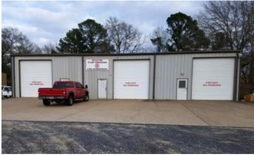
Figure 126: Flint-Gresham VFD, Station 2
